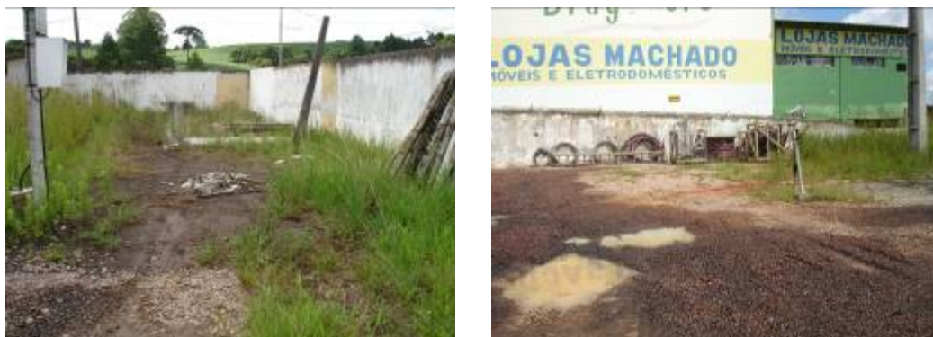
Figure 1. Mandirituba Power sub Substation
