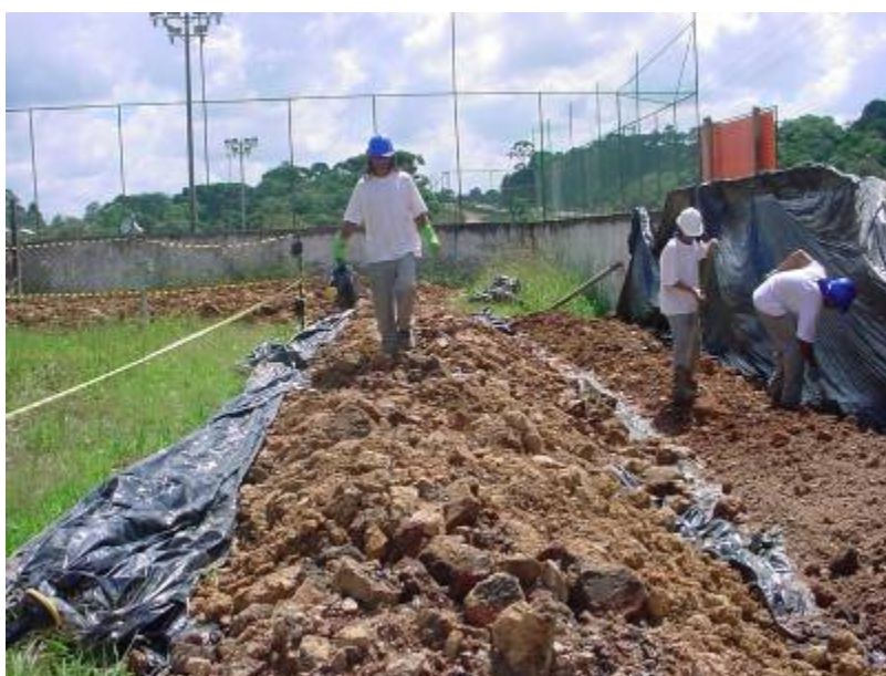
Figure 3. Remediation of the Mandirituba stacks.
