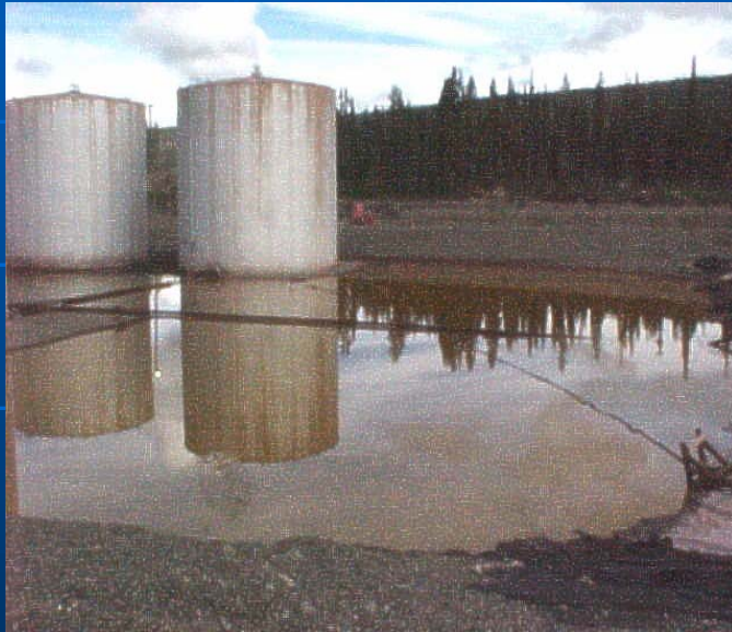
Before Spill Remed
