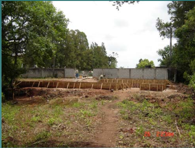
Canals under construction
