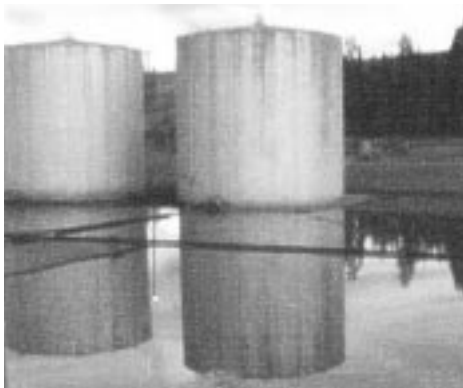
Spill after being sprayed with SpillRemed
